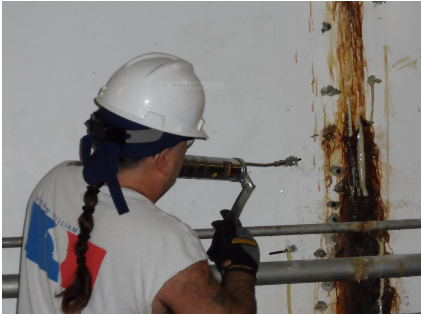
Sealing ground water leaks in the tunnel
